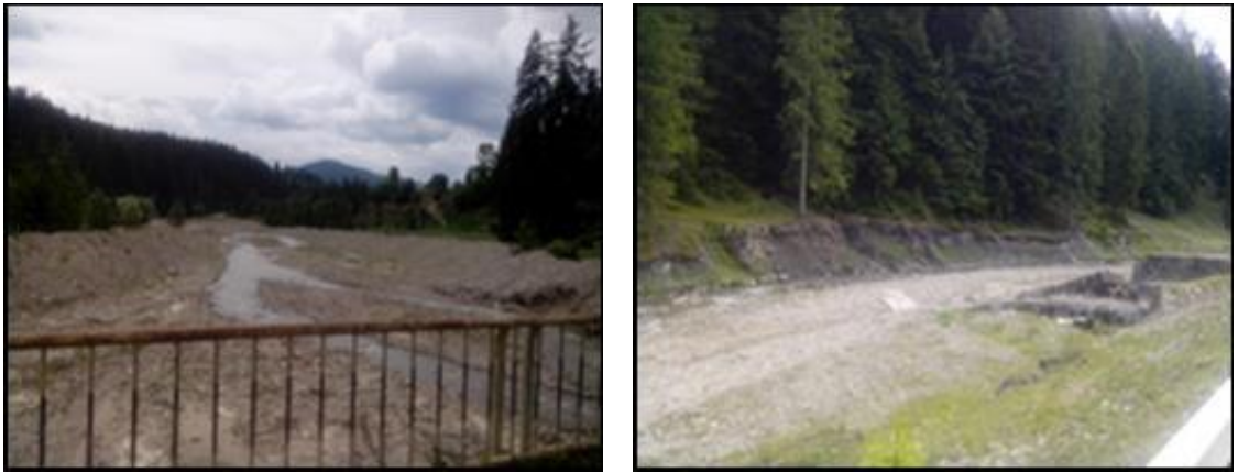
Figure 9a. Strengthening of river banks with sediment from embankment, b. The anti-erosion dam which was destroyed during the 2006 flash floods.
