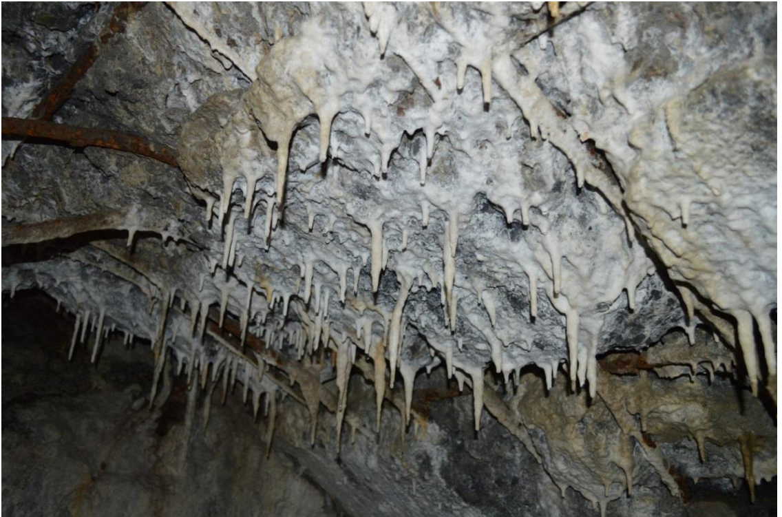
Figure 5- A group of stalactites on the ceiling of the bunker from Valea Teiului.
