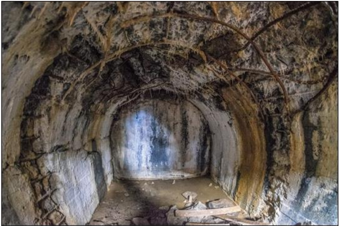
Figure 4 The interior of the bunker from Valea Teiului.
