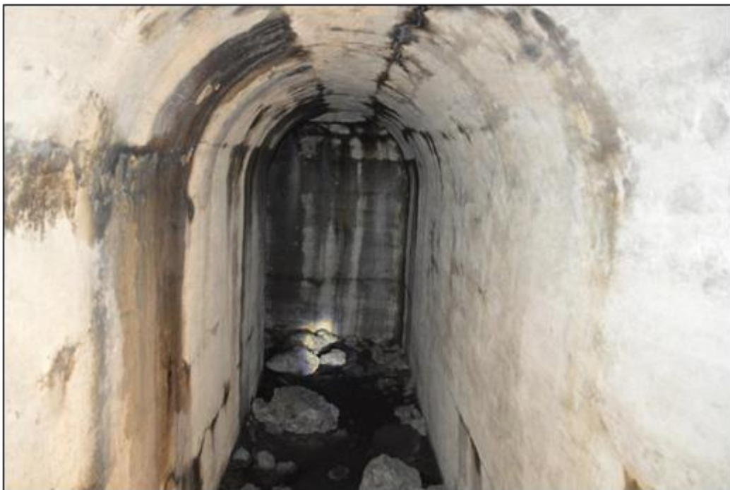
Figure 12 -Inside bunkers of Ilva Mică
