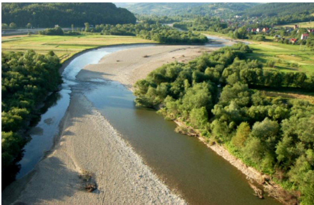
Figure 4. Oblique aerial photo of the Raba channel within the erodible corridor delimited in the vicinity of Lubień village. A relatively wide span between settlements and roads on both river sides provides the room for free channel migration and makes bank reinforcements unnecessary in this river reach. Photo by Łukasz Ślusarski, published by courtesy of Ab Ovo Association. This figure is available in colour online at www.georeview.ro
