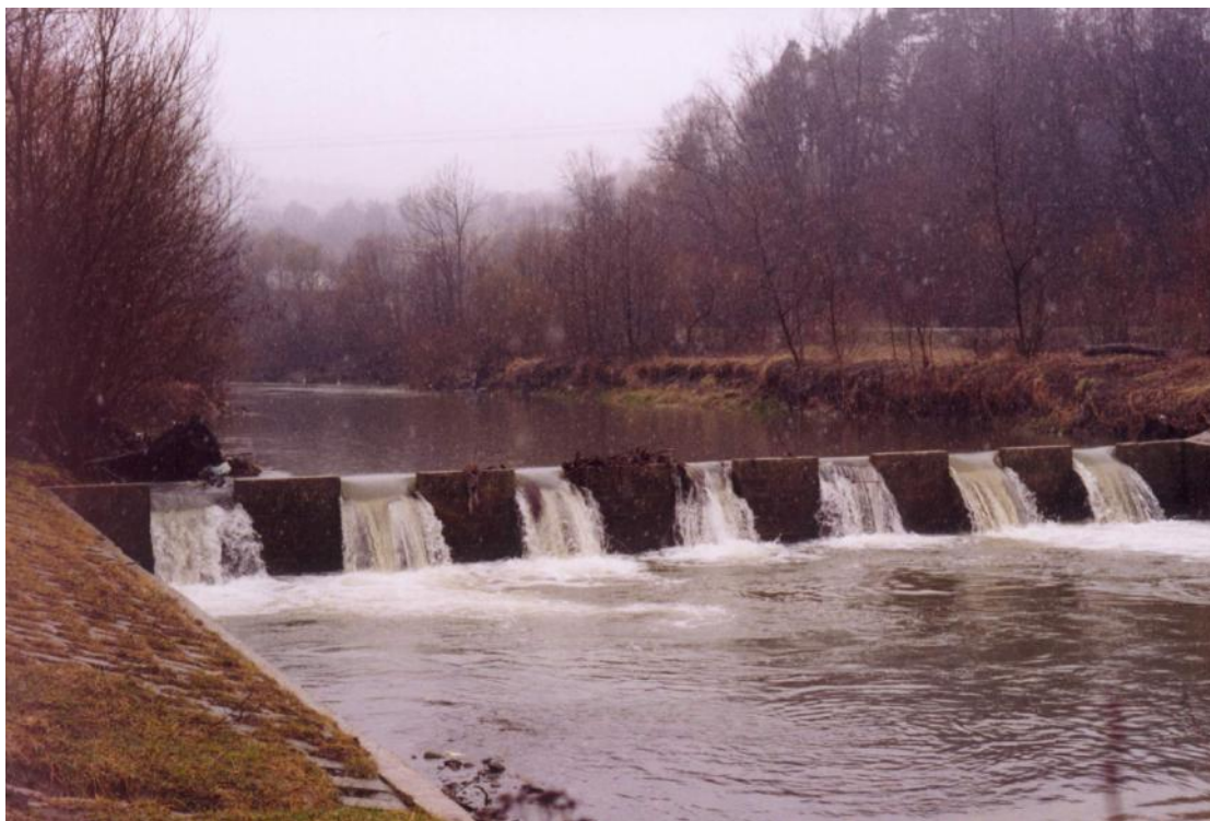
Photo 2. The piano-notch of the Kasinczanka drop hydraulic structure under bankfull.
