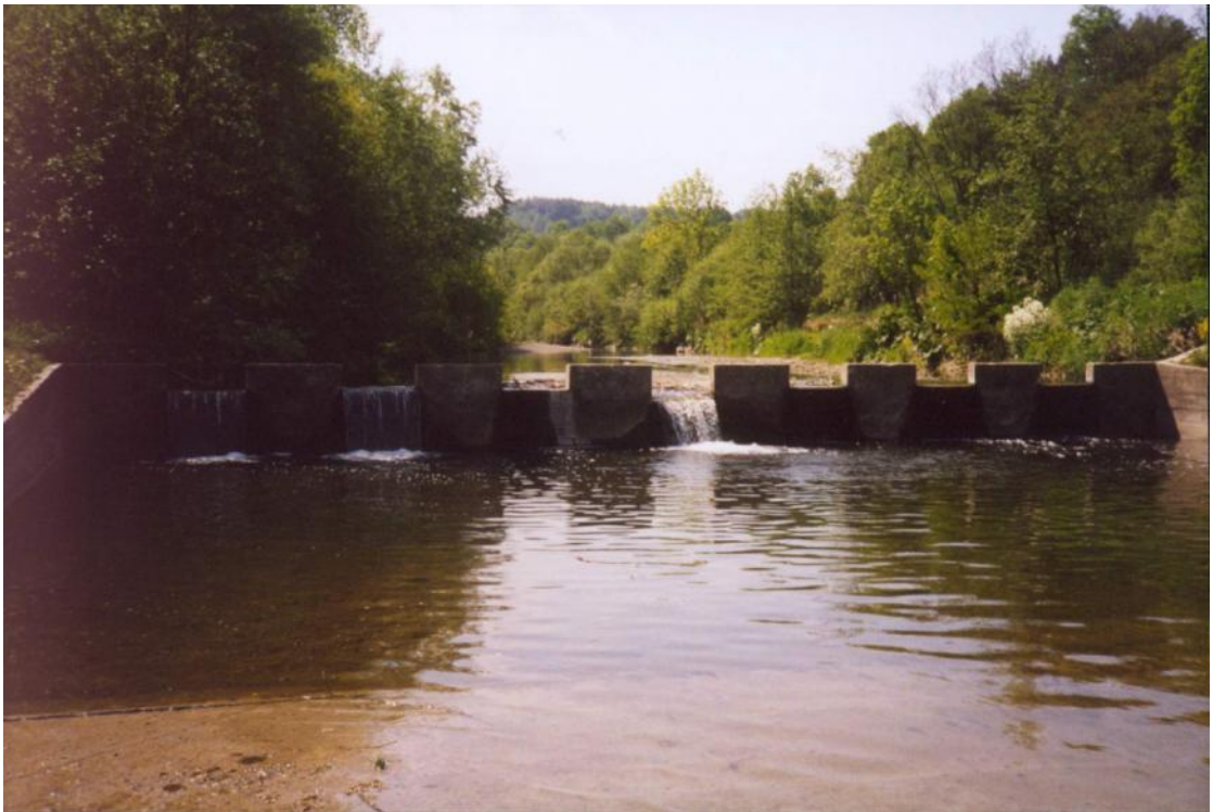
Photo 3. The piano-notch of the Kasinczanka drop hydraulic structure under low discharge conditions.
