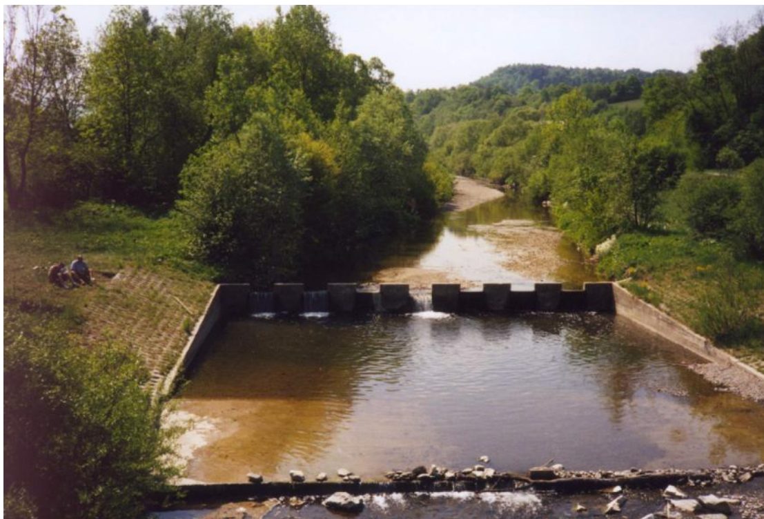
Photo 1. Drop hydraulic structure in Kasinczanka stream – general view.
