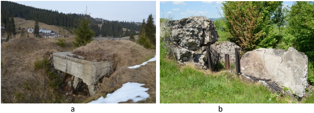
Figure 8 Concrete casemates at Tihuța Canton (Bîrgău Gorge, a), and Ponce Hill (Ilva Mică, b) ( source: the author ).
